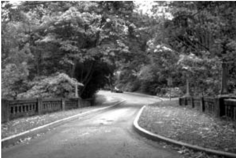
This choker on a two-way roadway in Seattle, Washington, narrows the street from two lanes to one. Traffic is forced to slow down and, in some cases, wait for an approaching vehicle to pass before proceeding.
