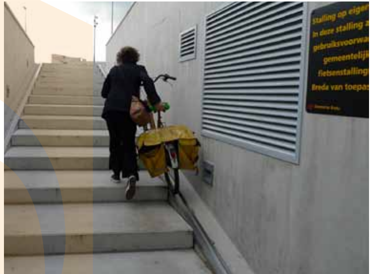
Stairs with a pair of concrete ramps in the Dutch city of Breda, south of Rotterdam. The gentle grade makes handling a loaded bicycle easier.
